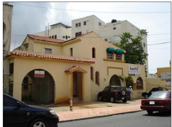
28) DR. DELGADO No. 1, SOLAR No. 13 DEF., MANZANA No. 399
