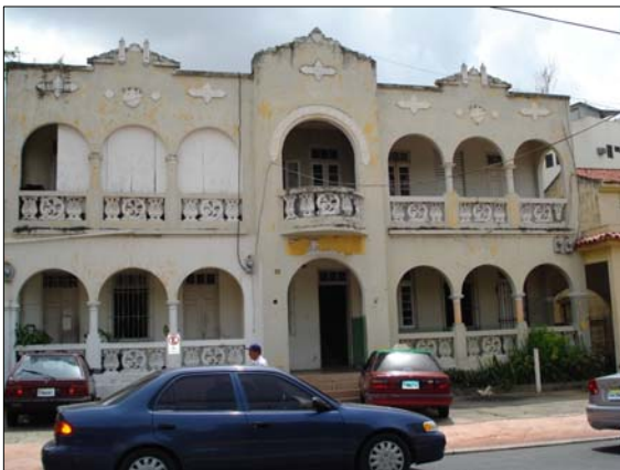
27) DR. DELGADO No. 3, SOLAR No. 14 DEF., MANZANA No. 399
